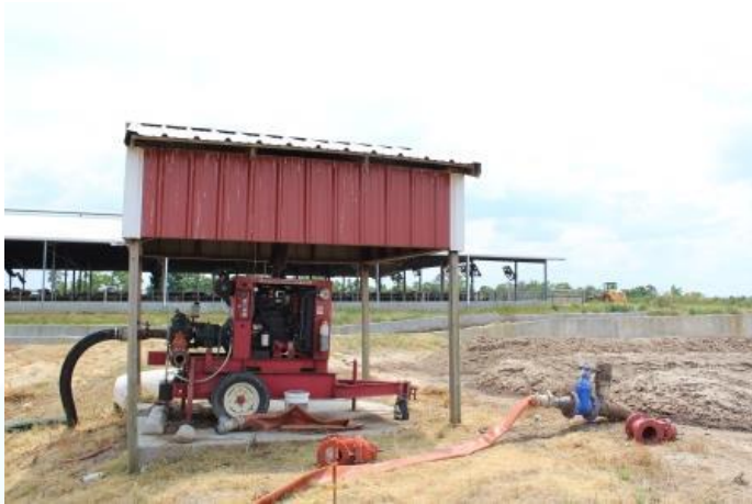
North Carolina Electric Cooperatives and White Rock Farms – Waste lagoon pumping system
